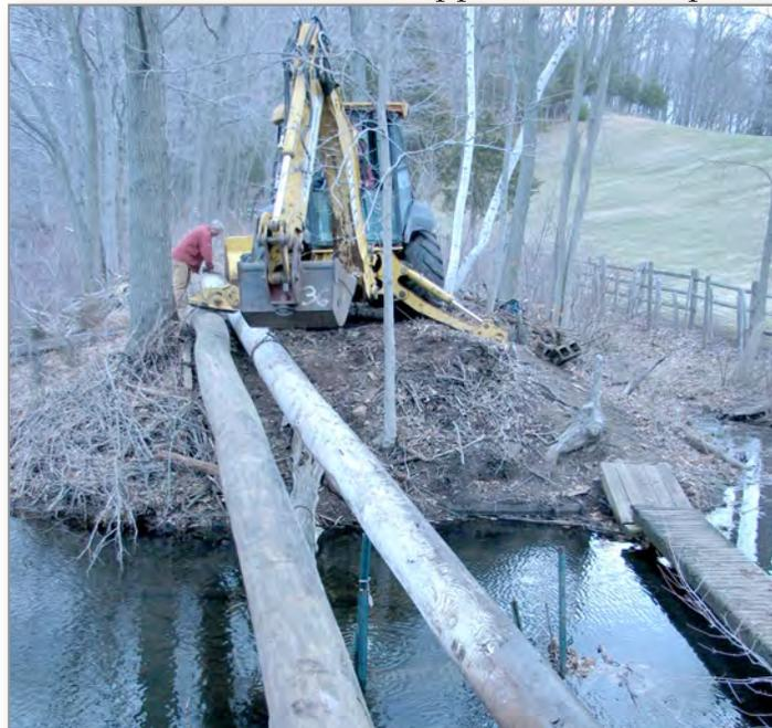
It was quite an undertaking, and the jockeying into place of these substantial supporting beams was quite a success. Hand rails and decking were installed later in the summer, and then a coat of redwood stain in the early fall finished the project.
